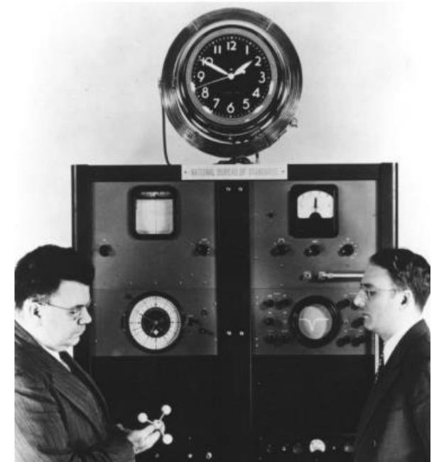
First "Atomic" Clock in 1949 ( \sigma \approx 2 \times 10^{-8} )
